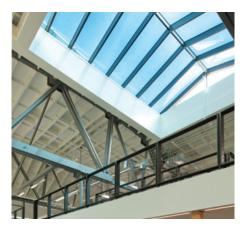
affecting workstations on the building's second floor. View Dynamic Glass was the chosen technology to control glare and minimize solar heat gain while still letting in the natural light people prefer.
