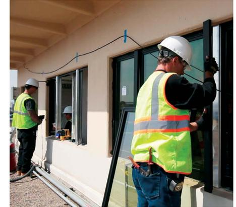
**Solution** The DoD replaced 1935 square feet of low-performing, clear glass with View Dynamic Glass. View worked with MCAS to develop an initial energy and benefits model. It showed that View Dynamic Glass enables a 23 percent reduction in HVAC peak-cooling load, a predicted 18 percent decrease in gas use and a 9 percent decrease in total energy use annually.
